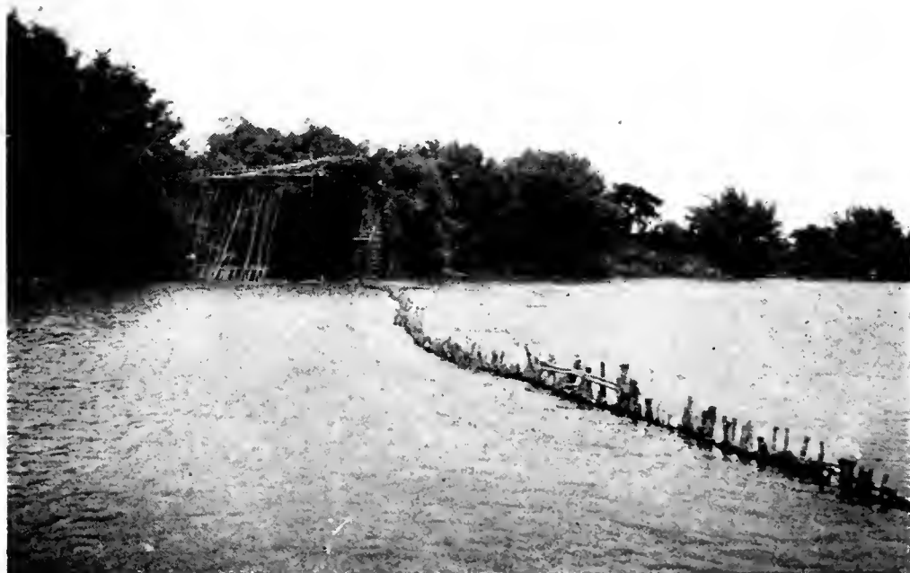
One wondered how these immense water-wheels that lift the rivers of Hainan into the thirsty rice-fields are put in position in a land of unassisted man-power
